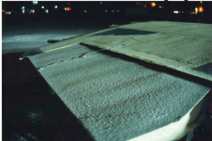
Photo 4.5 Snow Failure on the JetStar Trailing Edge
