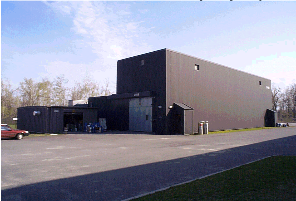
Photo 3.1 Outdoor View of NRC Canada Climatic Engineering Facility
