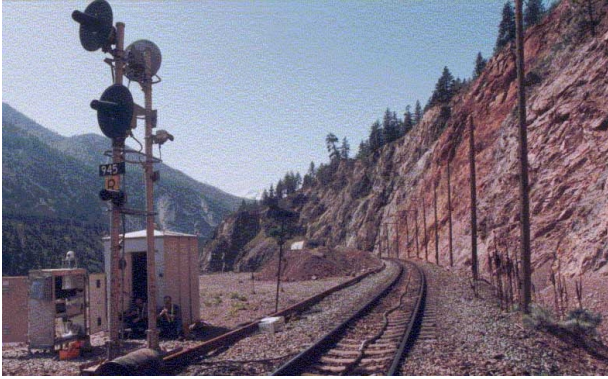
Figure 8 EMFD rockfall detection equipment at CNR Lasha. The protective conduit for the cable is visible between the rails at left.
