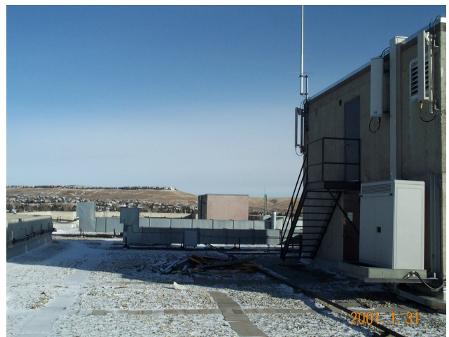
Photograph 4 - Fortress site (apartment building rooftop)
