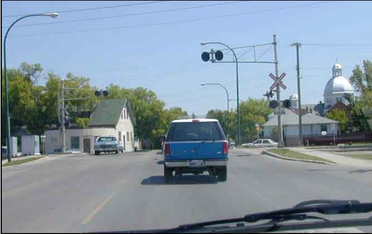
Figure 2.2 Crossbuck, lights on a pole and cantilevered over the roadway, 2-track sign and overhead lights in suburban Winnipeg.
