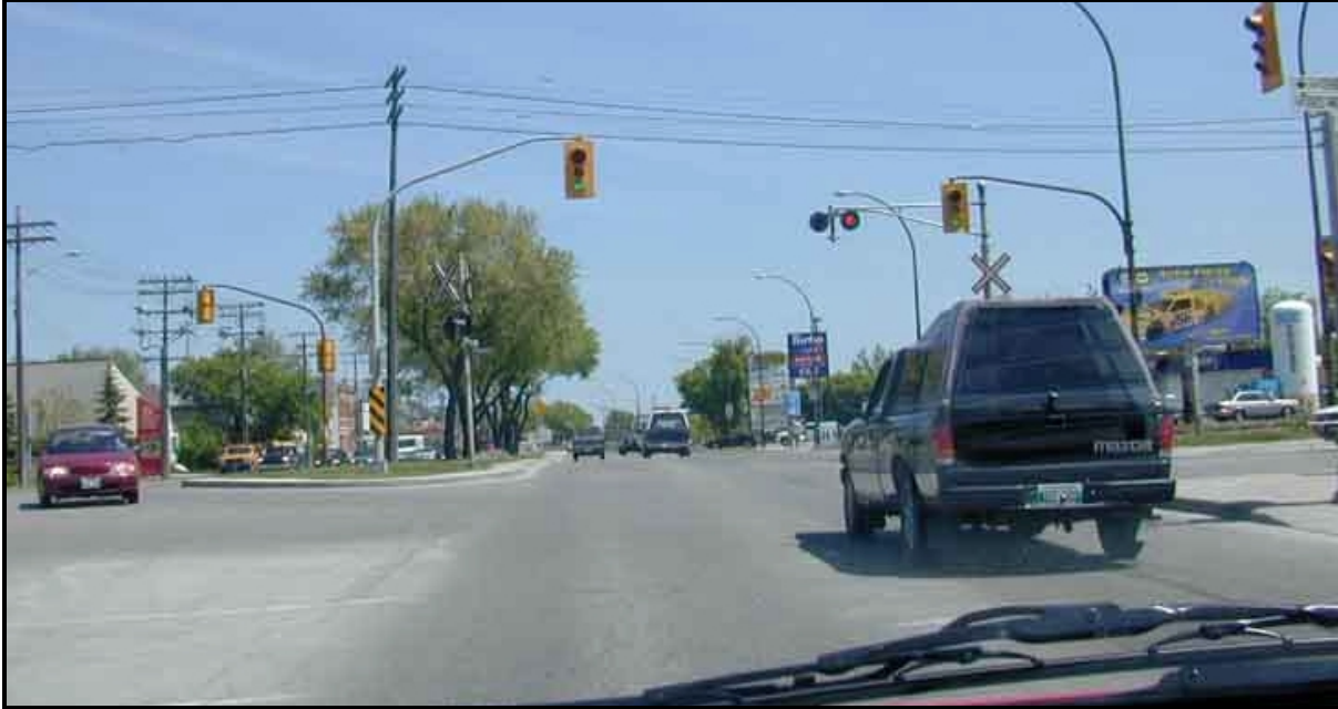
Figure 6.15 An intersection and a grade crossing in close proximity in urban Winnipeg. The visual demand of other vehicles, sign clutter, and signals make decisions to stop more difficult. The synchrony of the intersection lights (green) and crossing lights (flashing red) is not ideal. Interconnection of traffic lights and highway-railway grade crossing signals is suggested (Bremer & Ward, 1997).
