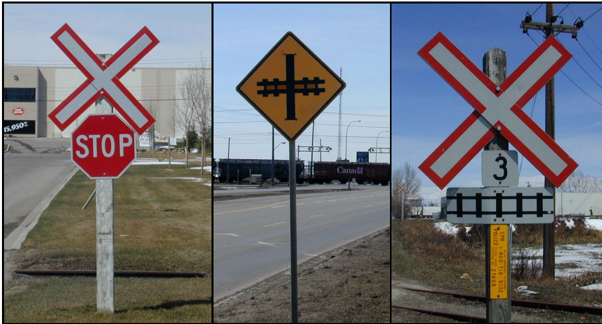
Figure 2.1 Advance Warning Signs: crossbuck (RA-6) with stop sign, advance warning sign, crossbuck with multiple track signage (RA-6s).
