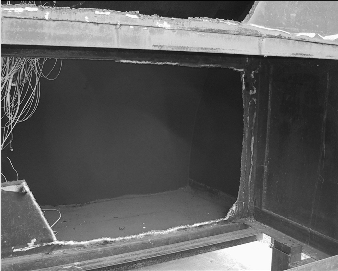
Figure 6: Back of Tank Wall
