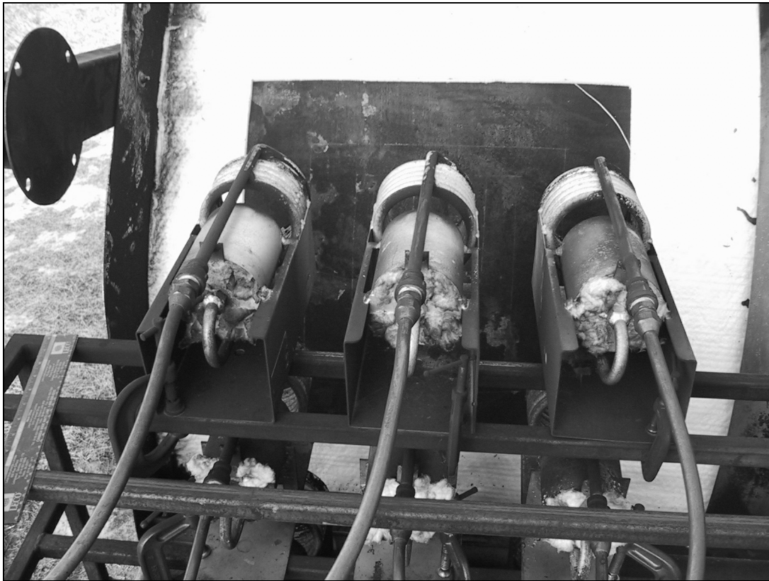
Figure 30: 61.0 cm Defect, Jacket Removed for Photo (Test 8)
