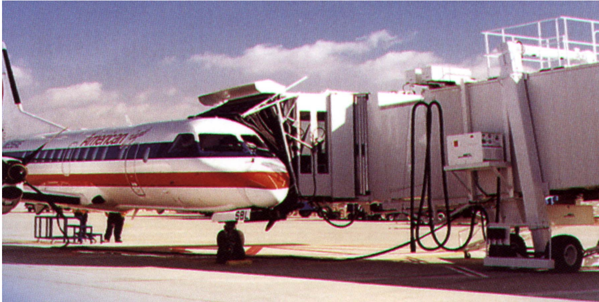
Photo G.4: Low-Level Boarding Bridge
