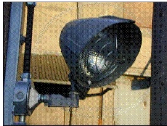
Figure 9 – Light pods after modifications
