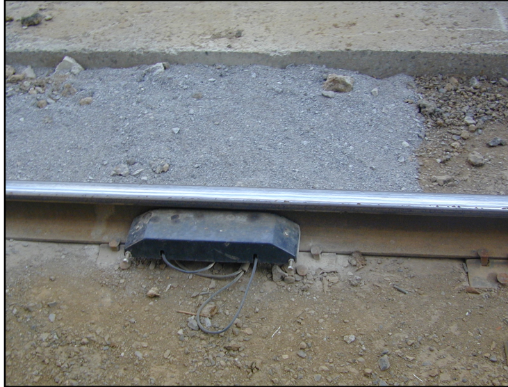
Figure 14 – A/B wheel sensor
