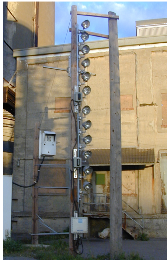
Figure 7 – Light pods after modifications
