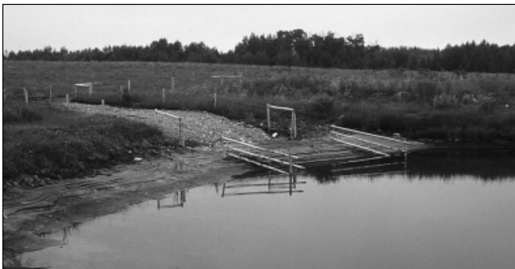
Access ramps must have a solid base.
