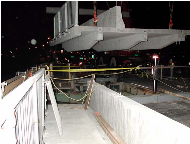
Fig. 7 – Installation of Approach span deck panel
