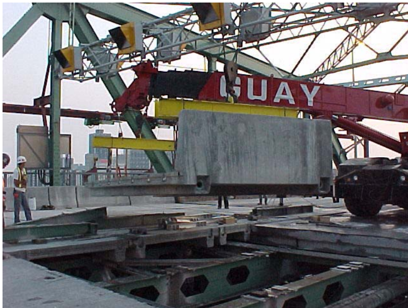
Fig. 8 – Installation of Seaway span deck panel
