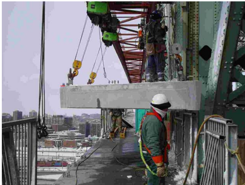
Fig. 10 – Installation of new precast bikeway panel
