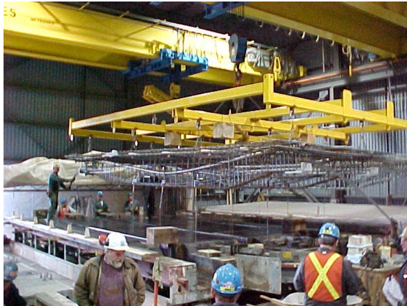
Fig. 6 – Fabrication of Approach span deck panel
