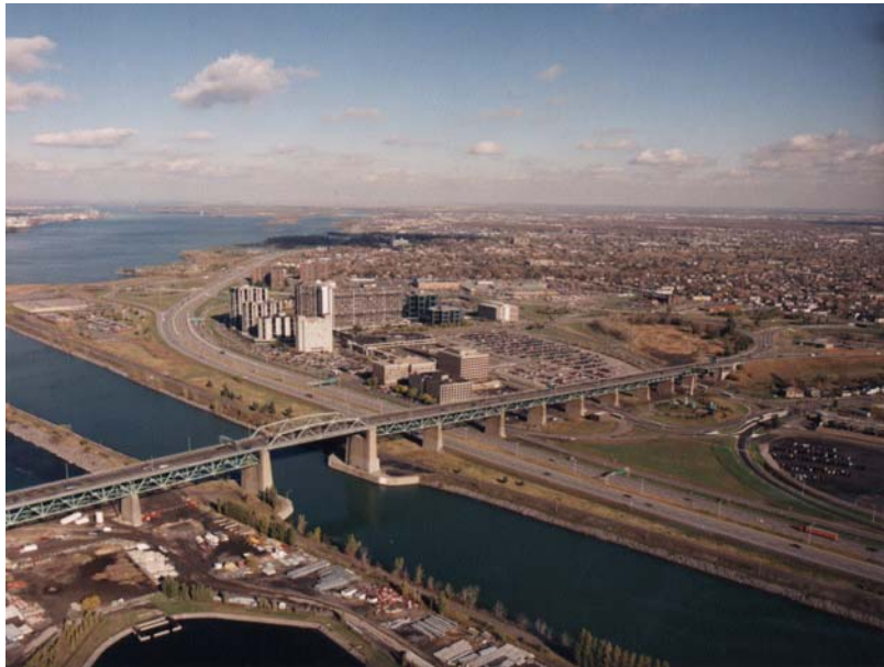
Fig. 2 – Seaway span and South approach
