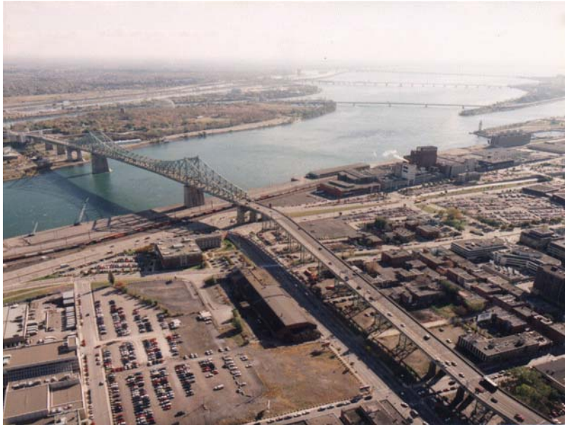
Fig. 1 – Main span and North approach
