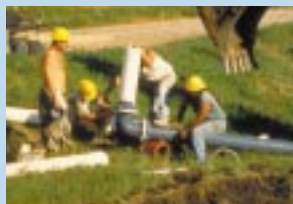
Installation de pipeline
