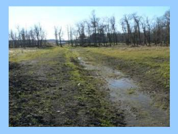
This photo depicts the drain path from the cattle containment area to the water holding pond. The main drain and drains within the cattle containment area have been fenced to eliminate any access by the cattle. The pond had to be constructed a distance away from the cattle area because of a high water table and soil conditions.
