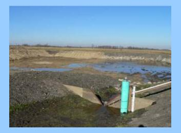
A holding pond was constructed to temporarily store runoff from a winter feeding area (field F6 MAP). The pond was designed to store approximately 75 mm of runoff from
