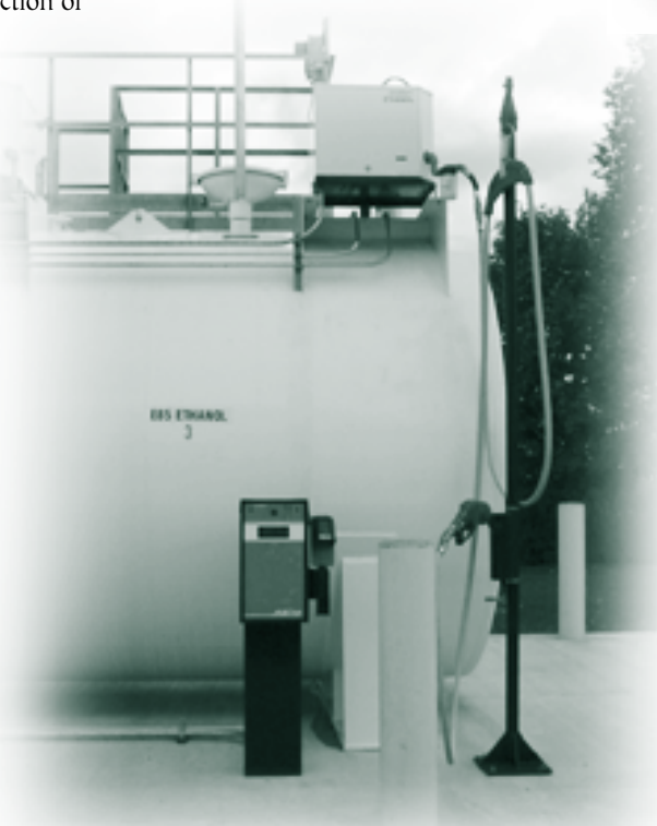
Agriculture and Agri-Food Canada in partnership with Natural Resources Canada, have developed new above-ground storage tank and supply/distribution systems suitable for oxygen-enriched fuels such as E-85.
