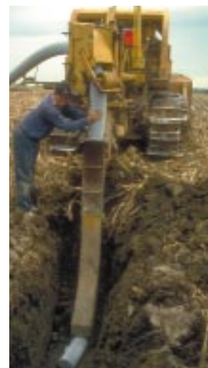
Laying drainage pipe
