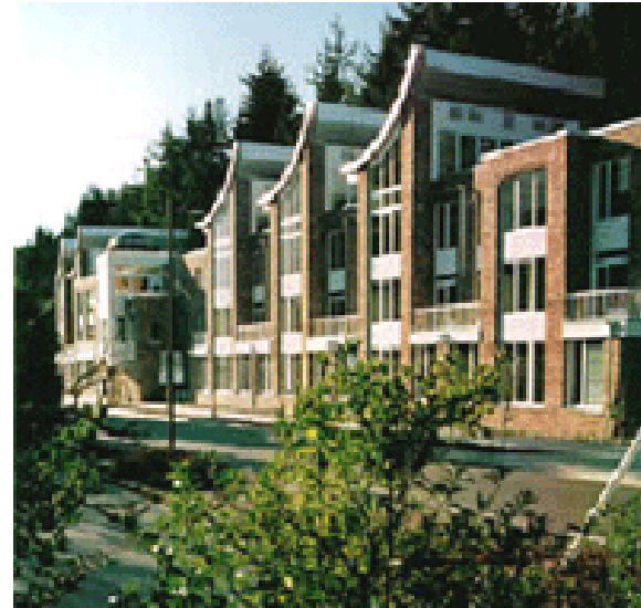
CK Choi Building (UBC): disconnected from the sanitary system.
