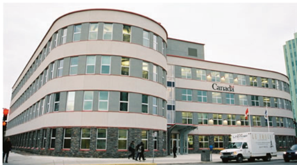
The Greenstone Building is the first North of 60 Leadership in Energy and Environmental Design (LEED)-Canada-Gold-Standard-certified office building. The building was completed and ready for occupancy in Fall 2005.
