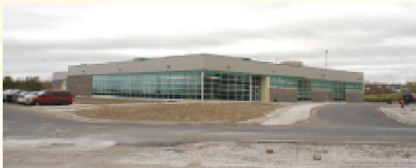
The Spiegel Tele-service Centre, as it stands today, up and running.
