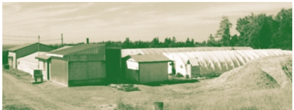
Denco Enterprises’ dry kiln and greenhouse complex. Biomass fuel is being stored outside on the right.
