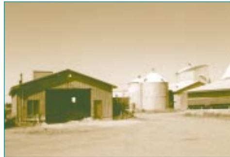
The Schurman Farm Ltd. Biomass Combustion System was constructed in the original farm workshop because of its central location.
