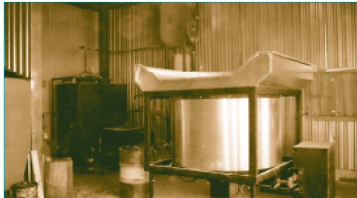
Valley Truss and Metal's 160-kW BCS with the new prototype round day bin designed for dry fuel.
