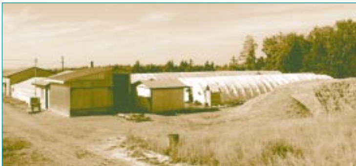
Denco Enterprises' dry kiln and greenhouse complex. Biomass fuel is stored outside on the right.
