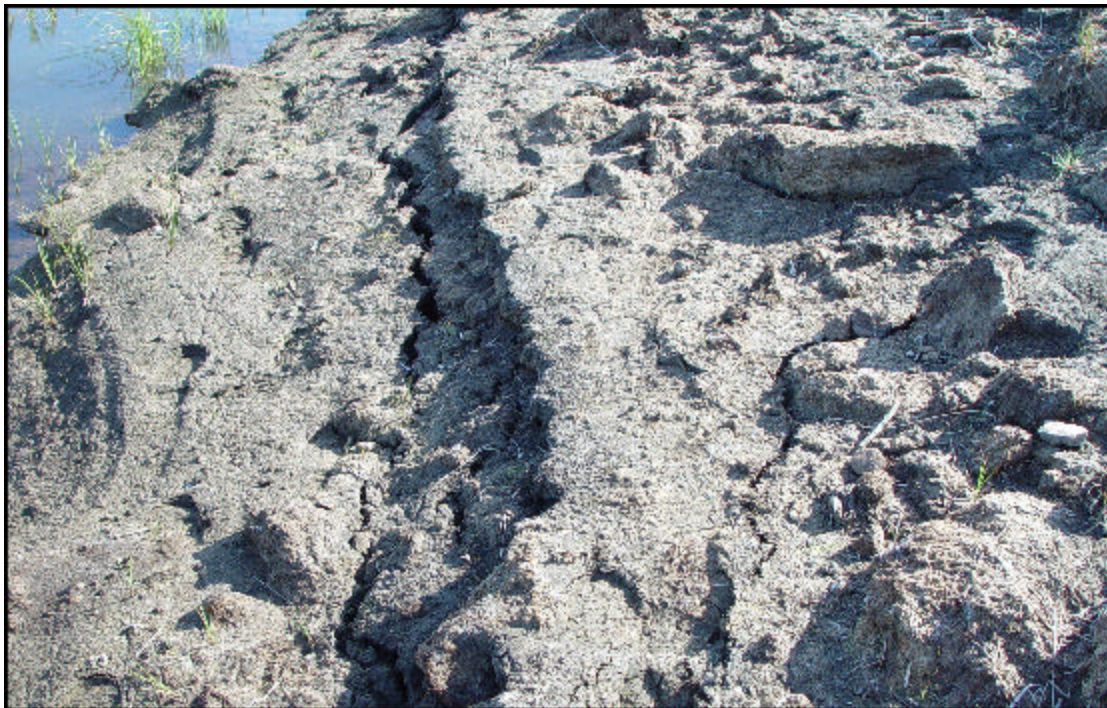
ESRF - M-15 - 0408210045.JPG - 69.081329466, -135.324234594 - Cracking/Sloughing, August 2004
