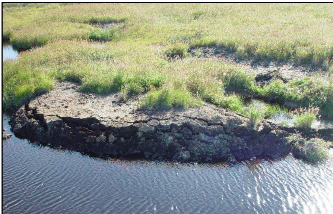
ESRF-P-53-0408210034.JPG - Sump sloughing/cracking around edge, August 2004
