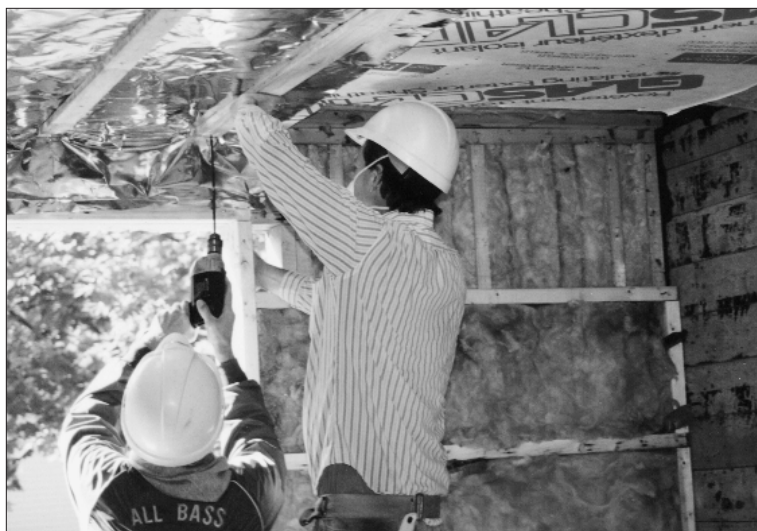
Reconstructing the ceiling and walls with aluminum foil over insulation
