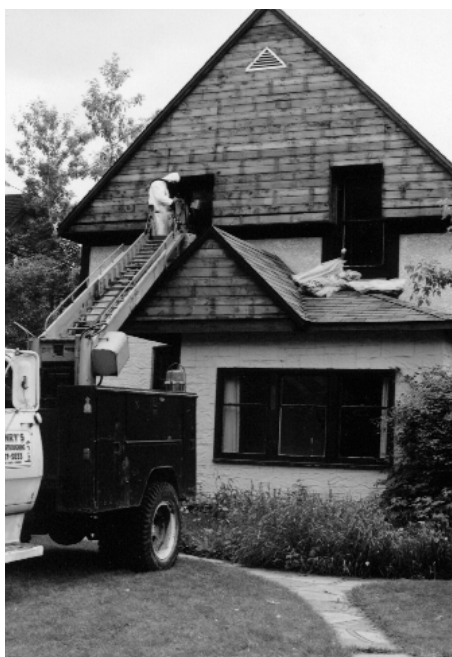
Before, in mid-renovation and after
