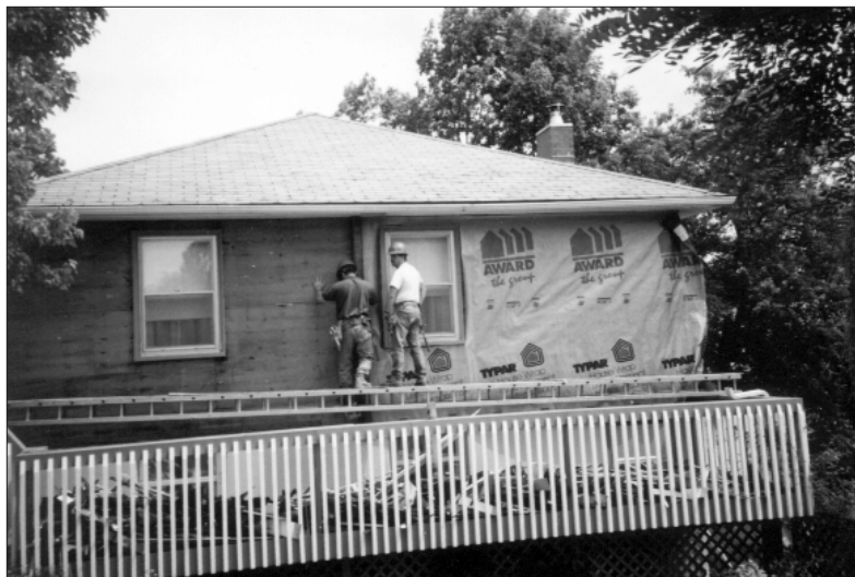
Exterior air barrier being installed
