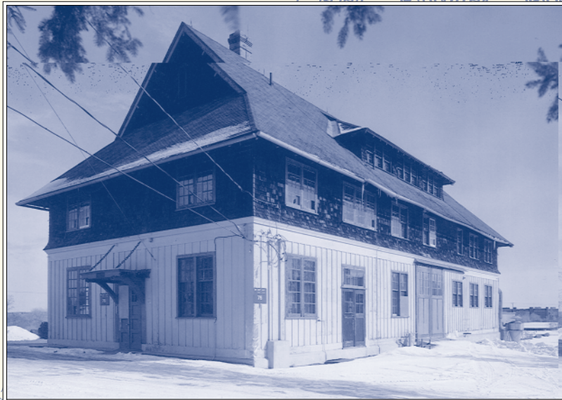
Cereal Barn Building, Ottawa, Ontario. (Heritage Recording Services, Parks, 1986)
