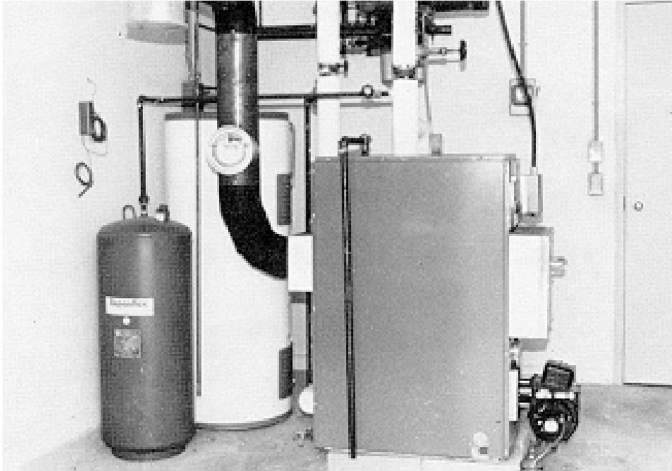
**Fig. 13 Oil-fired, hot-water furnace used as a source of heat for brooding either chicken or turkey broilers.**
