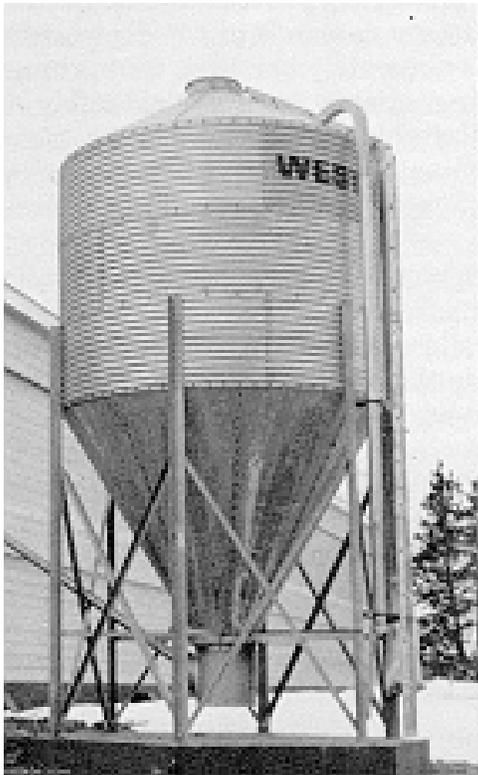
**Fig. 28** Corrugated metal, bulk feed tank with centre draw.
