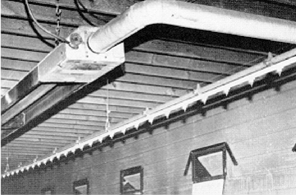
**Fig. 15 Propane gas-fueled radiant-heating unit for brooding either chicken or turkey broilers.**
