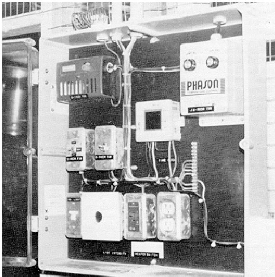
**Fig. 27 Panel for controlling photoperiods, light intensity, and air change. Containing metal box is equipped with a Plexiglass cover for dust- and water-proofing during wash-up.**
