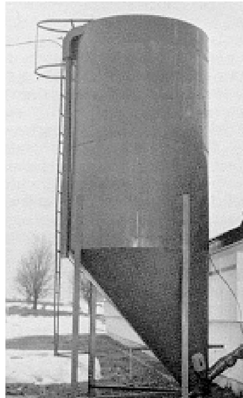
**Fig. 29** Welded steel, bulk feed tank with side draw.
