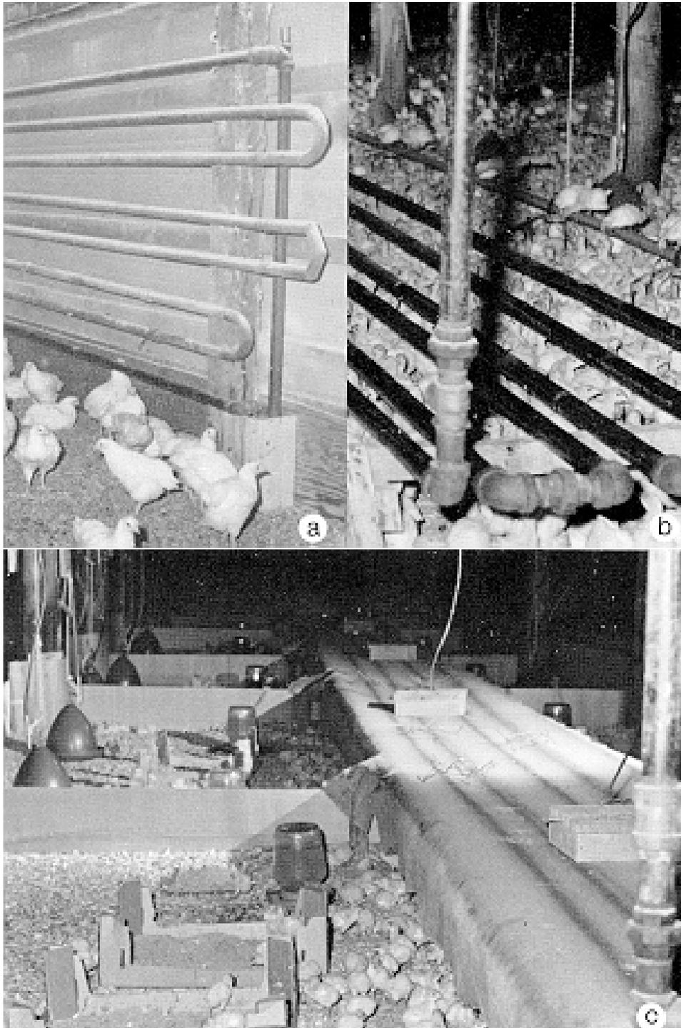
**Fig. 14** Hot water circulates through pipes to provide heat for either chicken or turkey broilers.
