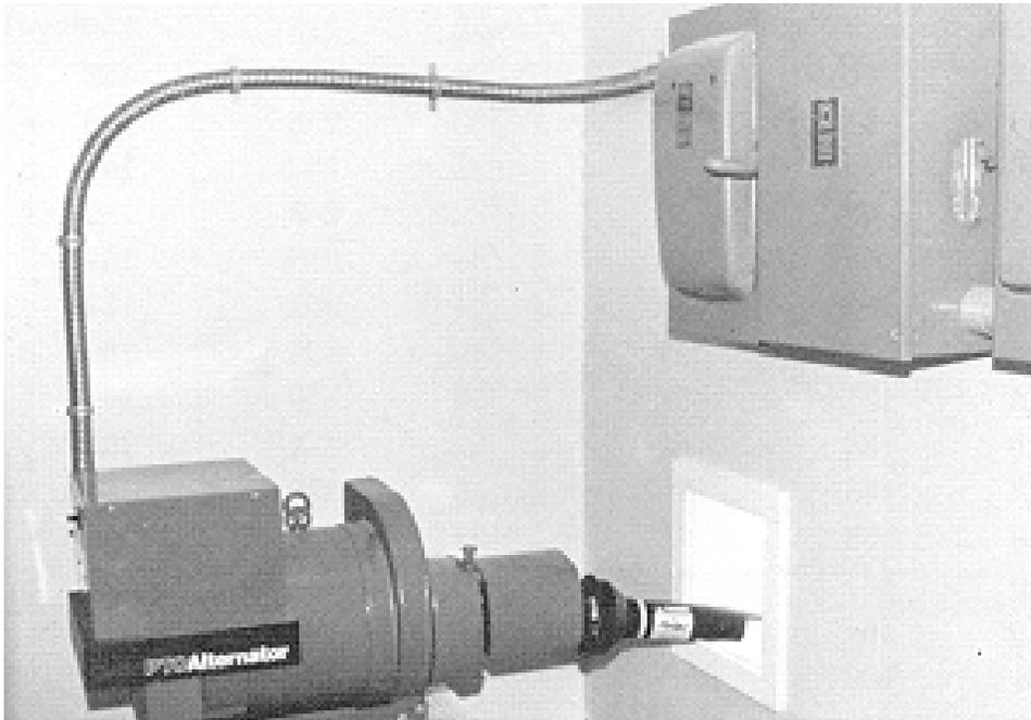
**Fig. 17** Stand-by electrical generator, which can be powered by hooking it up to a farm tractor in the event of a power failure.
