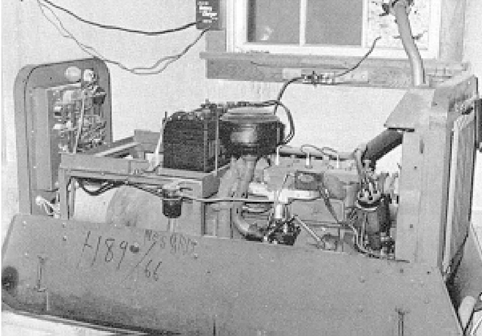
**Fig. 16** Auxiliary power unit used to provide essential electricity during power failures.
