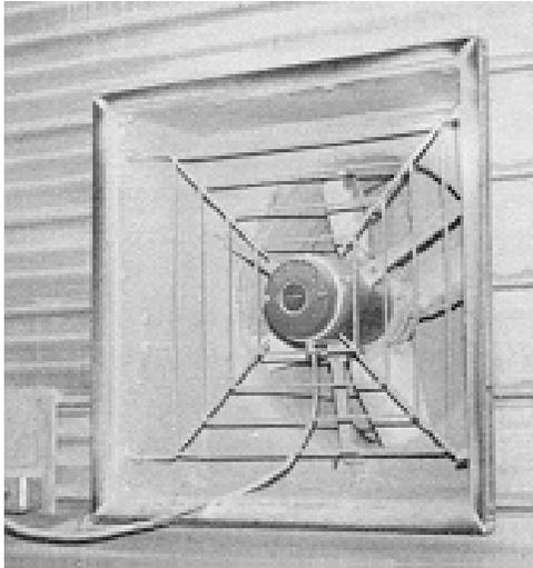
**Fig. 22** Fan used for exhausting air from broiler barn.
