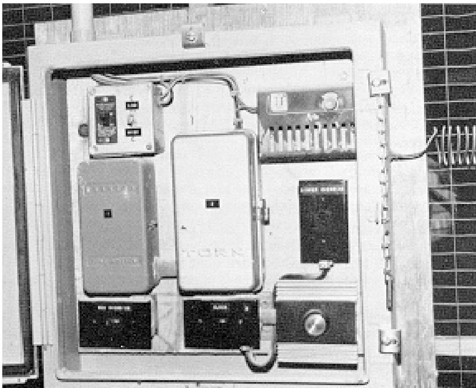
**Fig. 24** Ventilation and light control panel used in a brooder house.
