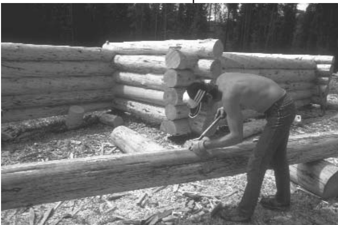
Building a log cabin, Yukon Territory.
