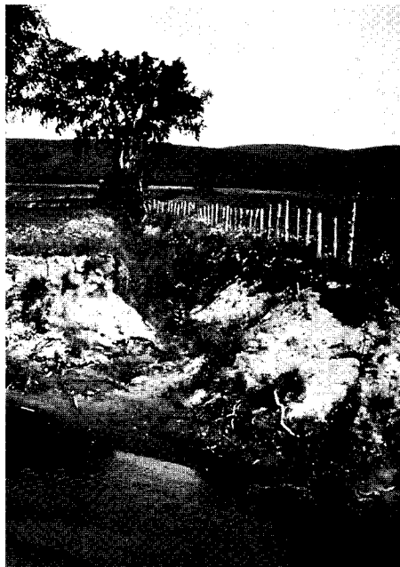
The eroding riverbanks are propitious to the waterways' contamination by farm pollutants.
