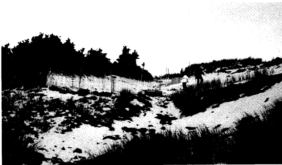
Dune restoration project, fence building at Pointe-de-l'Est (Magdalen Islands), summer 1996.
