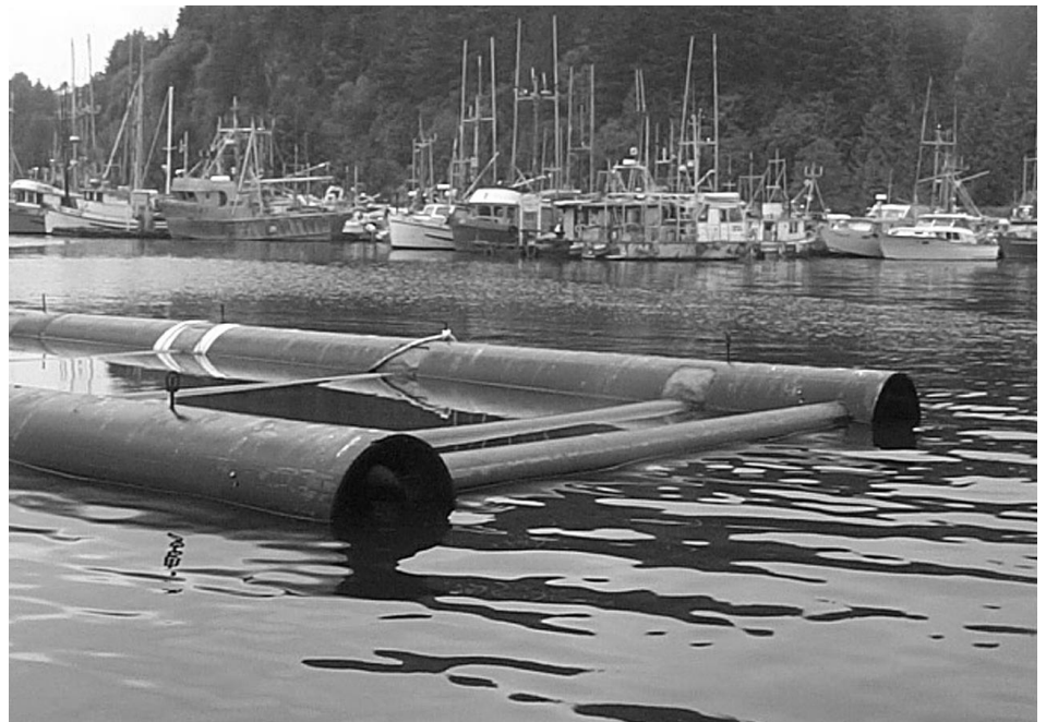
The 280-metre plastic breakwater moored at Prince Rupert's Rushbrooke site replaced a deteriorating log bundle breakwater that had lasted only nine years.
