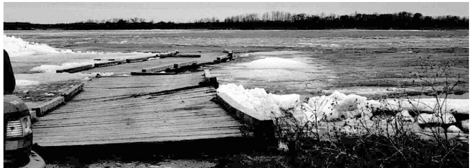
The wharf at Duck Bay before the Harbour Authority rebuilt it.
