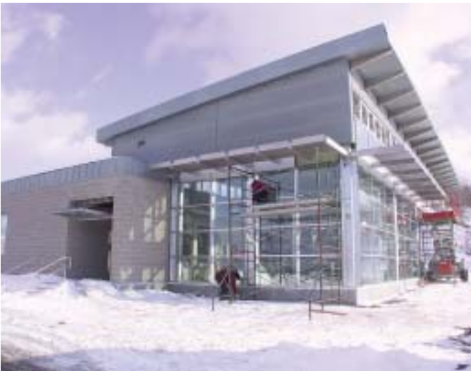
Energy Center Cooling Plant near completion.
