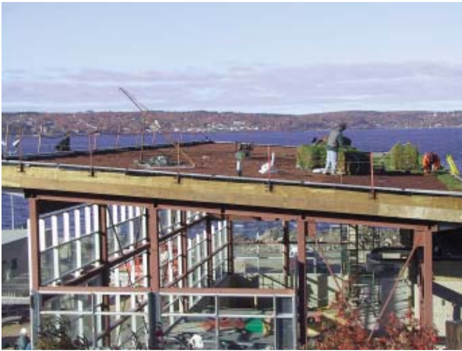
Installation of grass roofing material.
