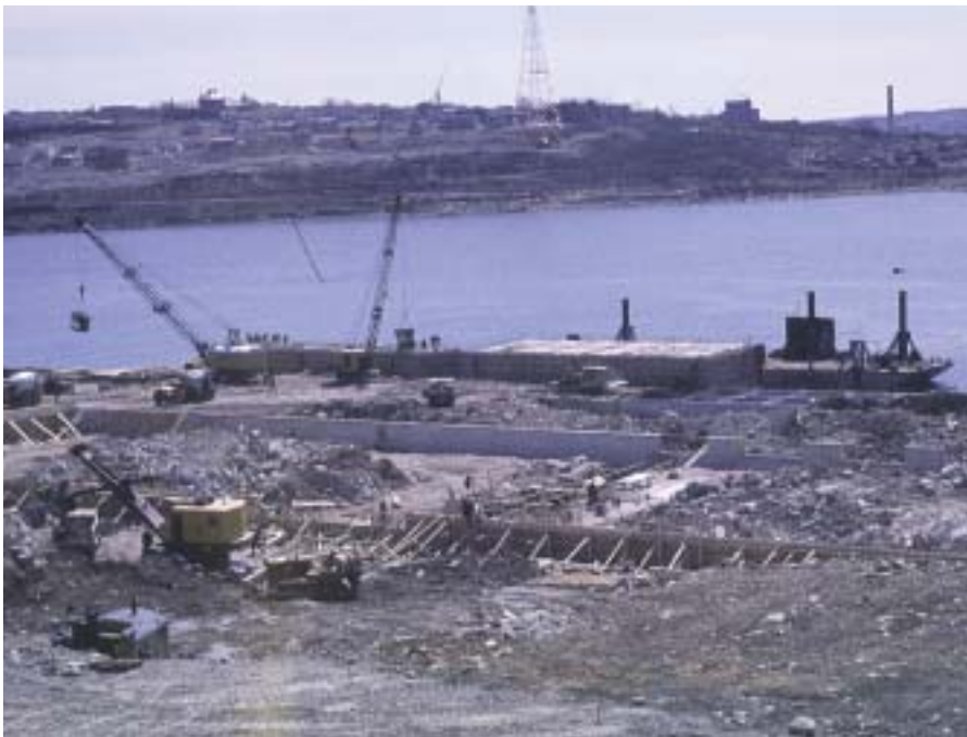
Construction at the BIO site, May 1961 – photo by John Lazier.
