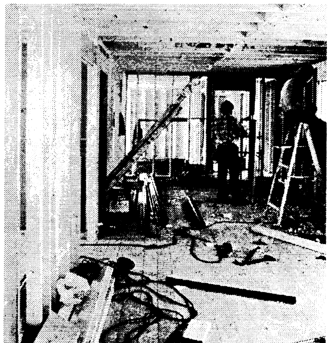
A typical woodframe house under construction
