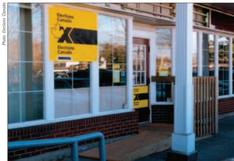
All federal polling stations and offices used by returning officers during an election must have level access. At the 2000 general election, returning officers modified many facilities (including the one pictured above) to provide such access.
