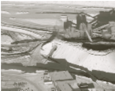
This coal-processing plant is located near a national park. This is an example of one of the types of natural-resource development activities occurring in close proximity to national parks.
