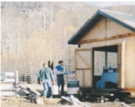
A work release crew works on the rodeo grounds near Grand Cache, Alberta.
