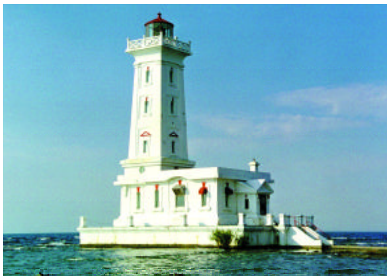
The Point Abino Light Tower, Lake Erie, Ontario, a federal heritage building
