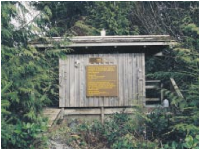
This composting outhouse in Pacific Rim National Park Reserve is virtually waste-free. In addition, its fan is solar powered P. Wilkinson
