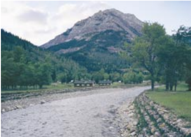
This stream has been modified to reduce flooding in a campground in Waterton Lakes National Park.
