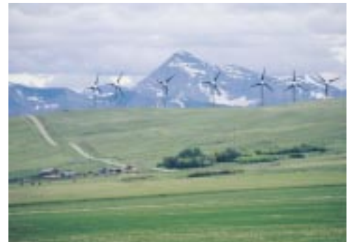
"Green" energy is available to some national parks, such as the electricity generated by these windmills near Waterton Lakes National Park. Blackbird Design
