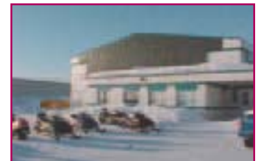
Alaittuq High School Solarwall
