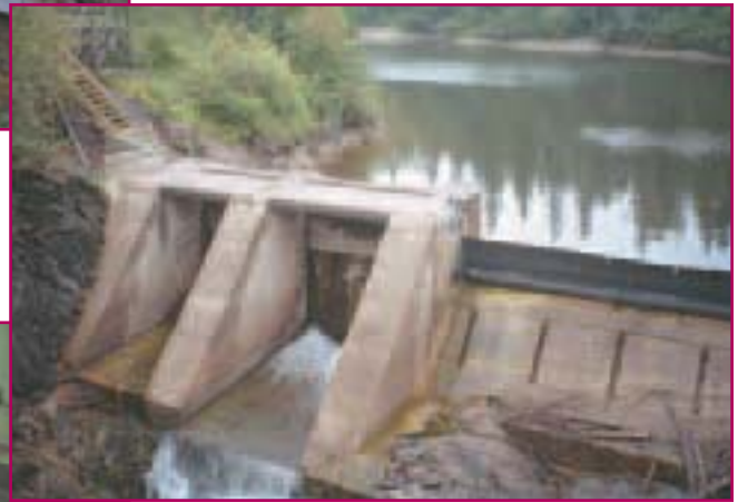
Black River Hydro Station
