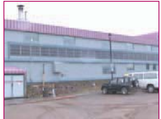
Solar panels mounted on the south wall of the Nunavut Arctic College
