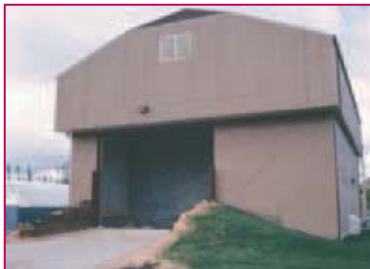
Community District Heating Plant
