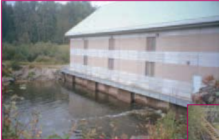
Black River Hydro Station
