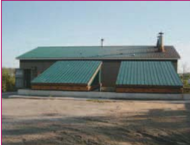
Community Wood Boiler Building
