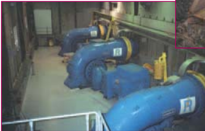
Black River – Penstock
