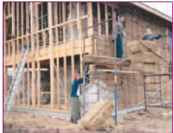
Kanata Healthy House Under Construction
