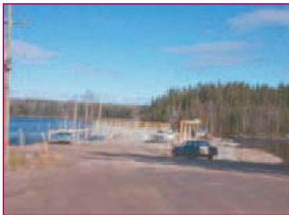
The Hydro Generating Station on the Severn River
