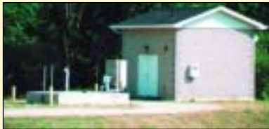
Sewage Pumping Station
