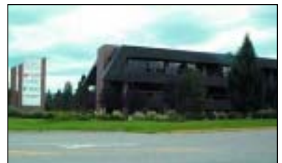
Westbank Administration Building
