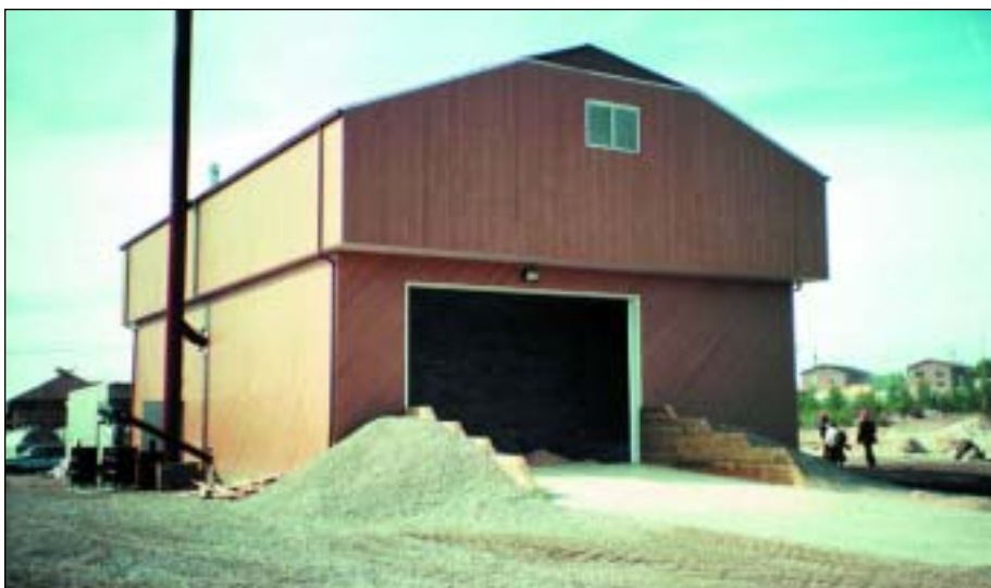
Community District Heating Plant
