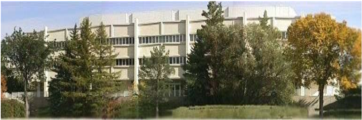
Laboratory Building (Departments of Biology, Chemistry and Biochemistry, Physics)
