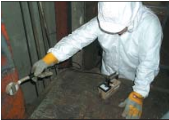
Other historic waste sites requiring remediation by the Office in 2000–2001 included this Toronto area building. Work was completed within CNSC deadlines.
