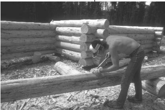
Building a log cabin, Yukon Territory.
