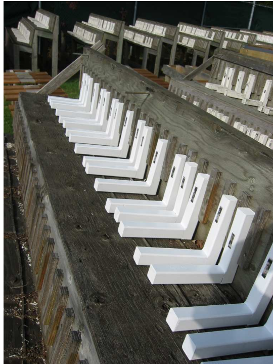
Figure 2. General appearance of L-joint test in field exposure at set-up.
