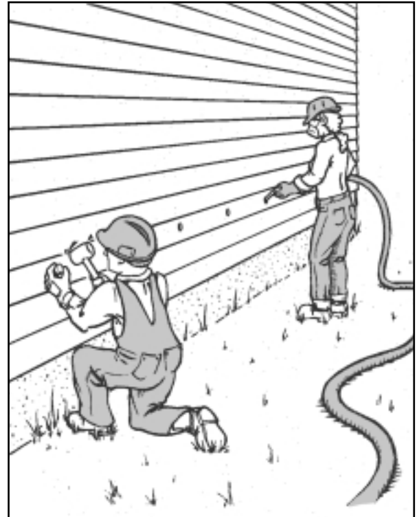
Blown-in insulation
