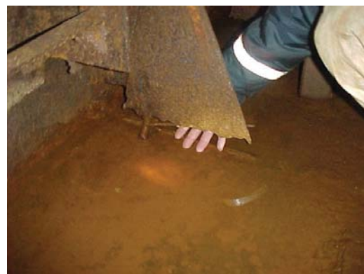
Corroded/Detached Bracket
