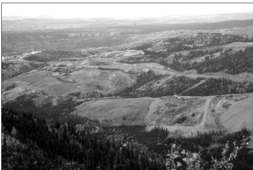
Figure 3. Recontoured open pits at the Brewery Creek minesite. Photo from Karen Pelletier.
