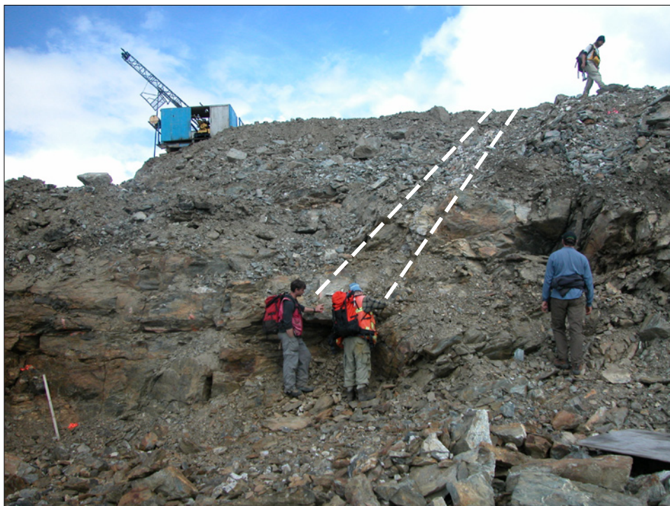
Figure 19. Portal site at Regal Ridge. The southwest vein is visible in the trench face (dashed line indicates zone).
