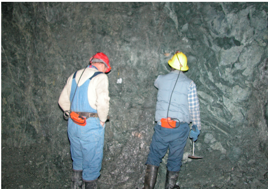
Figure 14. Quartz-sulphide mineral vein exposed in the underground extension at the Skukum Creek property.
