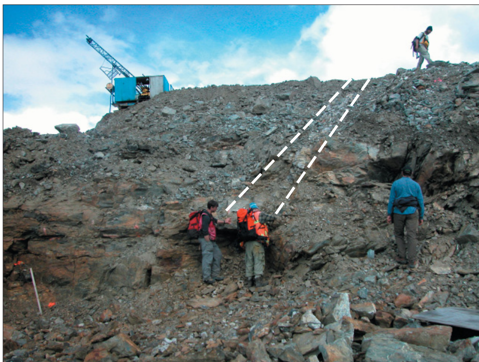
Figure 19. Portal site at Regal Ridge. The southwest vein is visible in the trench face (dashed line indicates zone).
