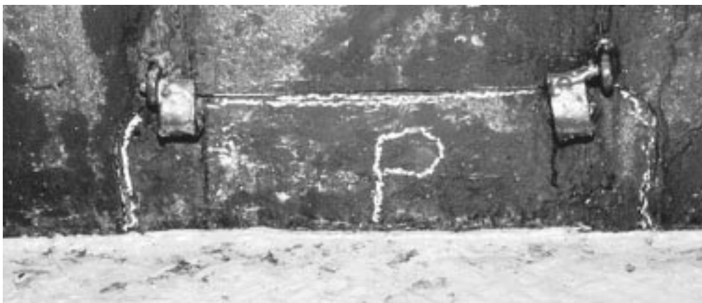
Main deck freeing port welded shut. Starboard side is similar.
