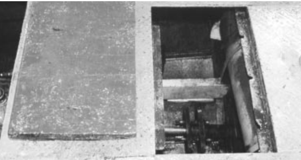
Hatch opening in main deck with no sealing gasket or means of securing flush wooden cover.
