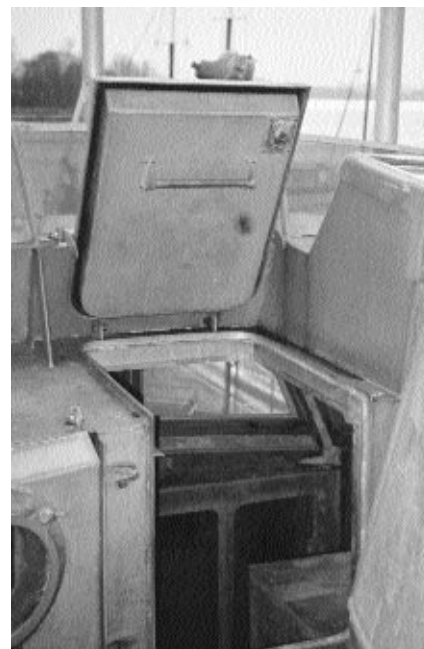
A combined hinged hatch cover and door on the centreline at the after end of the wheelhouse
