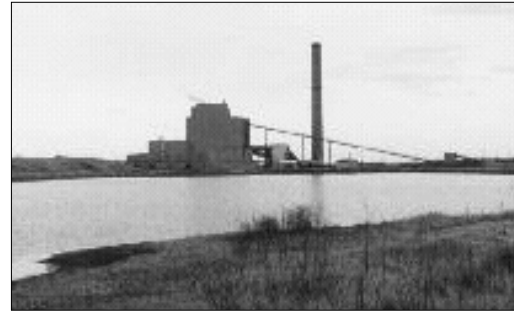
TransAlta Keephills, courtesy of Curtis Englot
