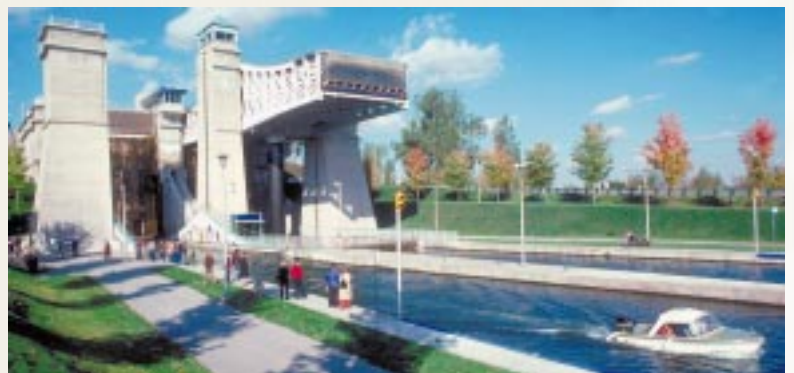
Peterborough Liftlock, Ontario World's Highest Hydraulic Liftlock (1896-1904)
