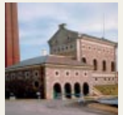
Hamilton Waterworks, Ontario Italianate Structure by Thomas C. Keefer
